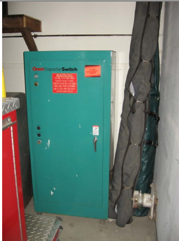
Photograph 16 - Transfer switch behind tanker
